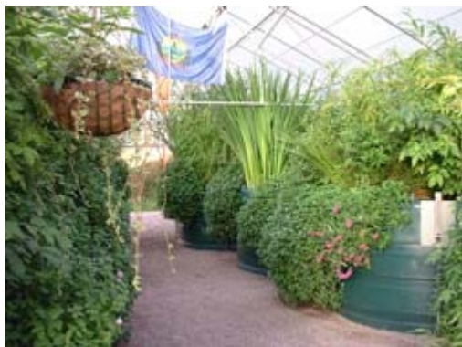
Living ecosystems treat wastewater on-site to meet state standards for discharge or reuse.
