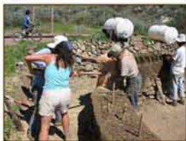
"Building with cob as a community"
