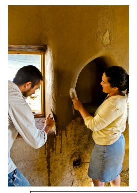
In this six day cob workshop, we focus on the characteristics of the natural materials most commonly used in construction: clay soil, sand, and fibers. Our main focus will be cob, though we will touch on various other building techniques that utilize the same materials, including adobe block, light straw-clay, wattle and daub, and plasters.
