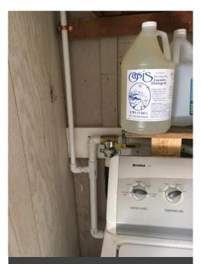
The laundry to landscape system starts at the washer with a three way valve, connected to the washer discharge tube, the sewer and the greywater lines to the landscape.
